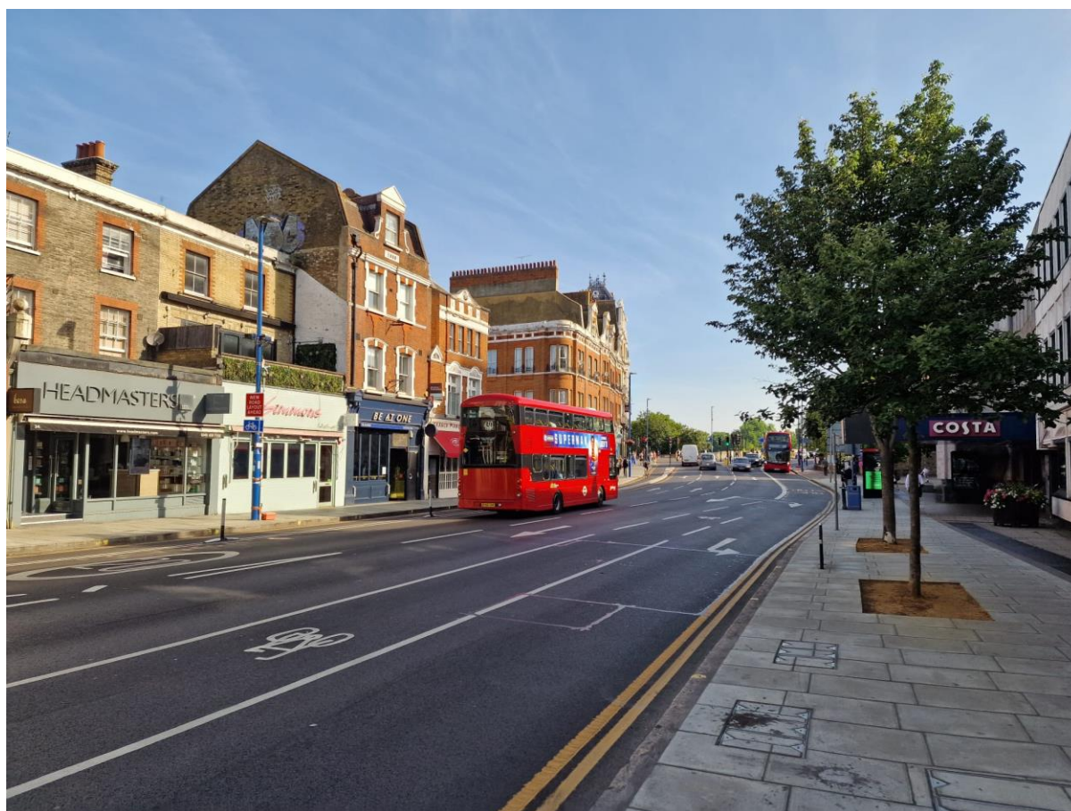
Figure 5-5-5 - Unsaturated pockets between Putney Bridge Road and Lower Richmond Road junctions with Putney High Street. Image points northbound.
