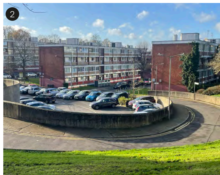
2 View into the site from Roehampton Lane
