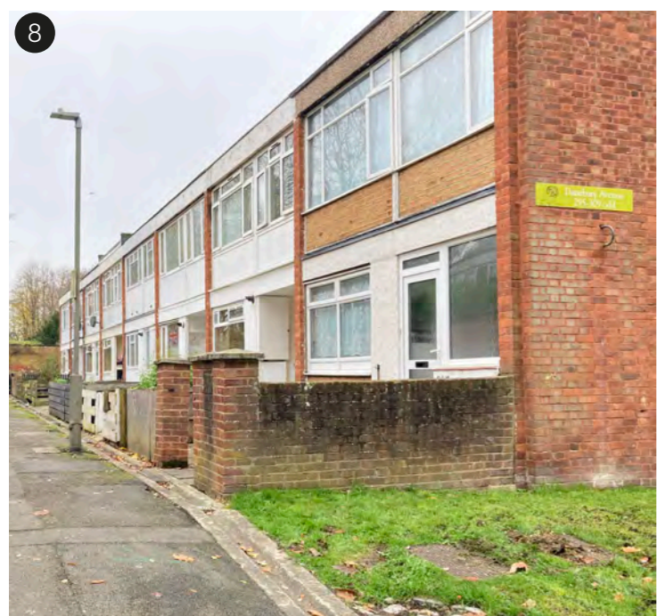
8 Two storey housing on the southern side of Danebury Avenue
