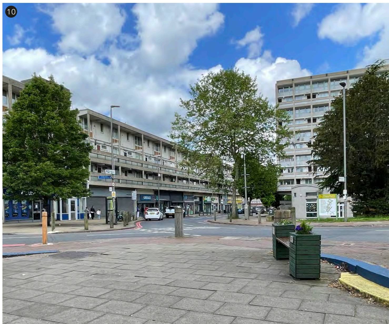
10 Local centre looking towards Allbrook House and Danebury Avenue
