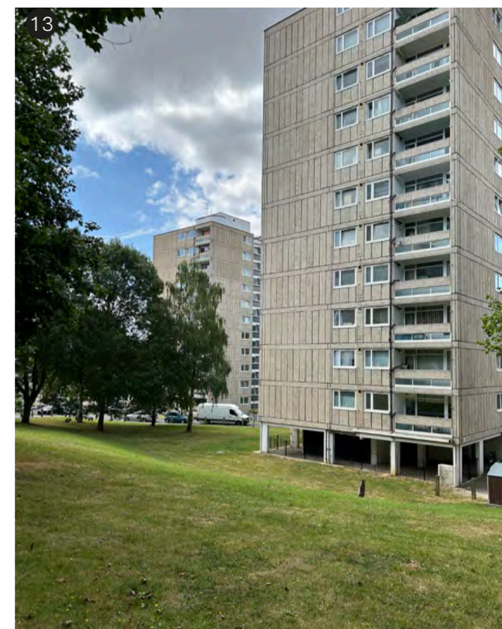
13 Tangley Grove Estate point blocks
